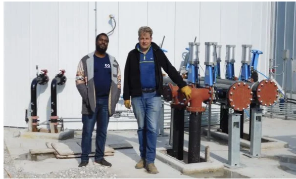
A Unique Bioenergy Project Fueled By Food Waste Powers Community Connections
